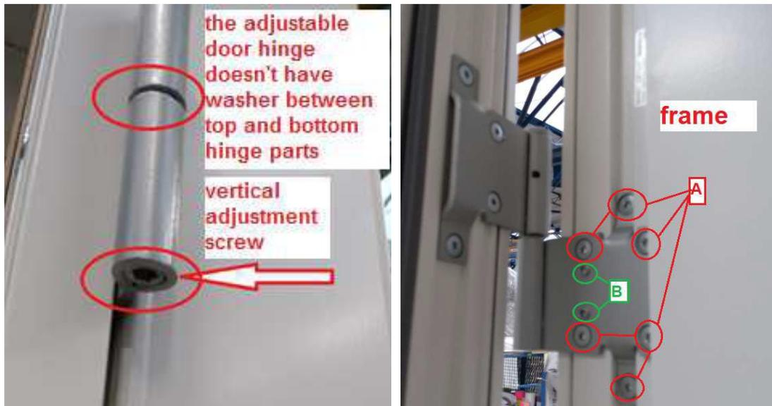
The green marked hinges on the top diagram including the vertical adjustment screw (+ /- 2mm) as shown on the left picture above. The hinges can be also adjusted in horizontal direction with using of screws marked with letter **B** on the right picture above.
